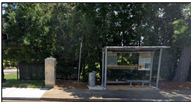
Figure 5: Example of a Designated Microtransit Stop
