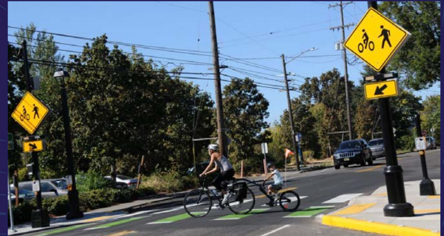
RECTANGULAR RAPID FLASHING BEACONS
