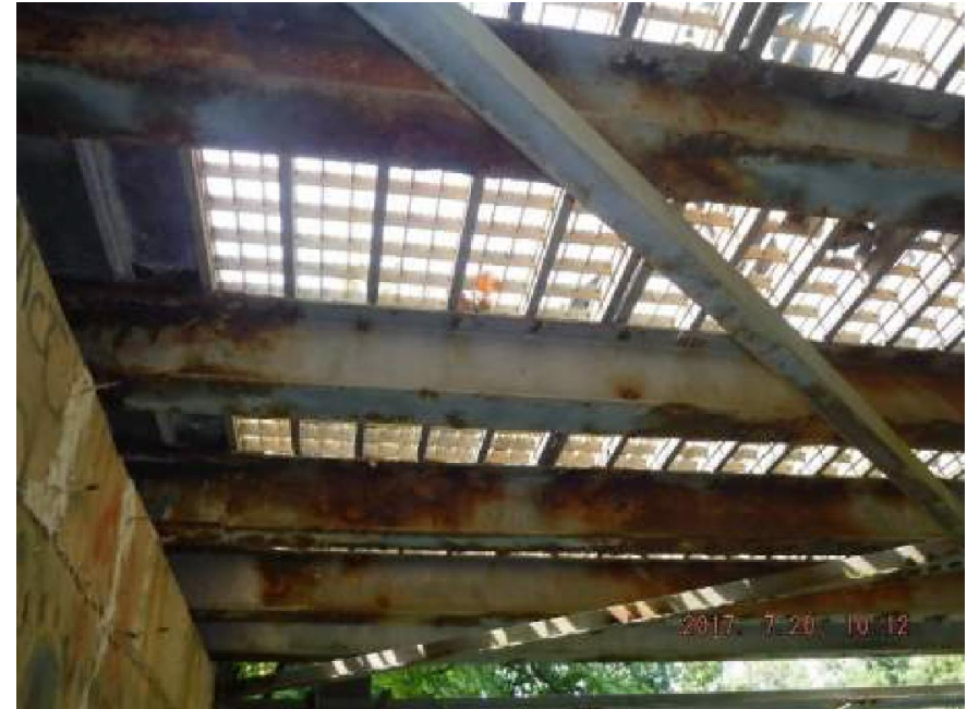
Corrosion and Section Loss – Stringers
