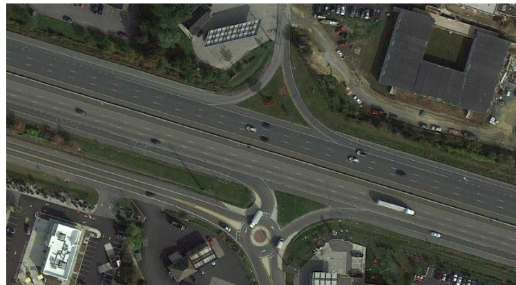
US 50/301 with Thompson Creek Service Road and Thompson Creek Road
