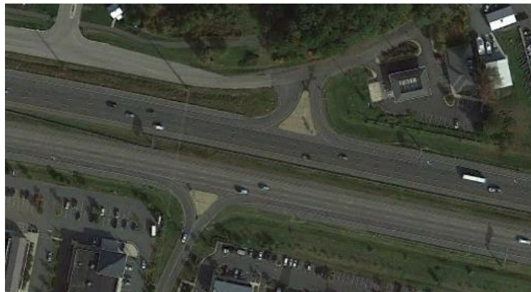
US 50/301 with South Piney Road and Piney Creek Road
