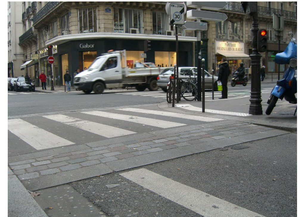
A raised crossing at sidewalk-level across a low-speed, low-volume street. Photo: Vladimir Zlokazov
