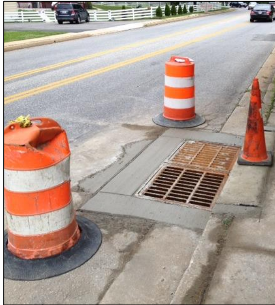
FY15 Award: $50,000 Baltimore County Storm Grate Upgrades
